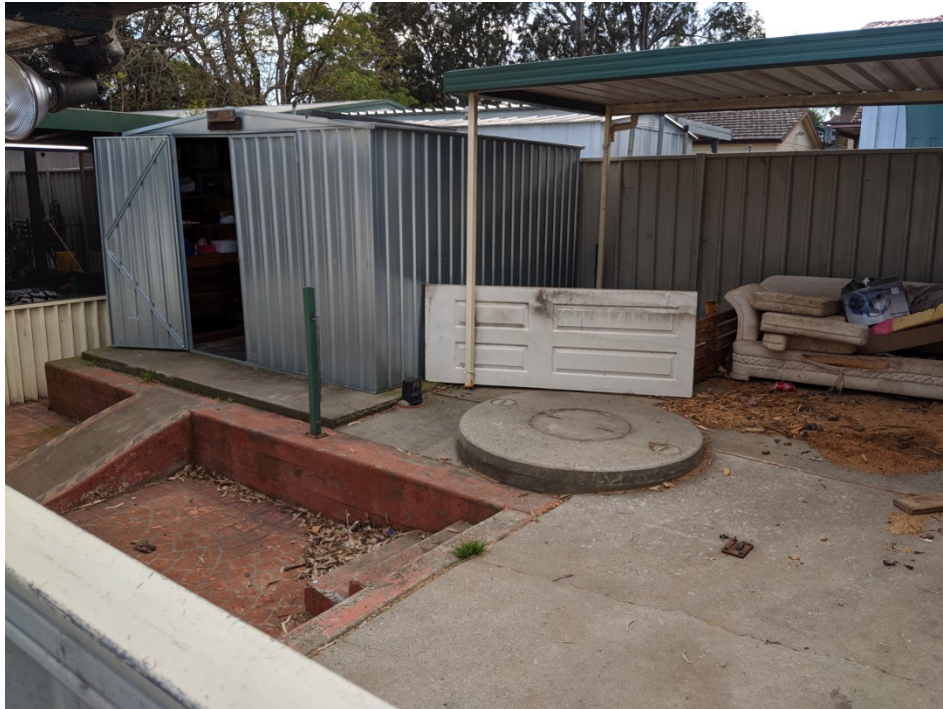
Photograph 3: Possible covered septic tank next to the house, in the eastern portion of the site (121 Minto Road).
